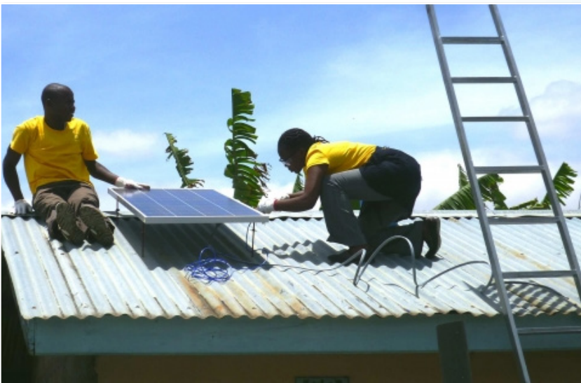
Installation of Solar energy
